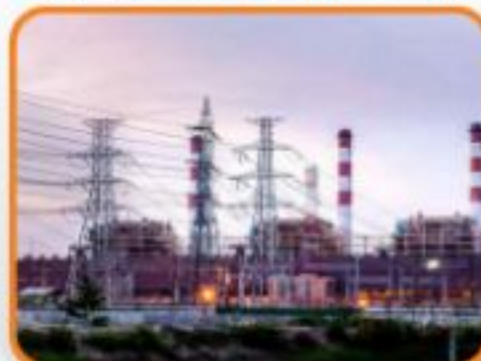
Power Generation, Transmission & Distribution
